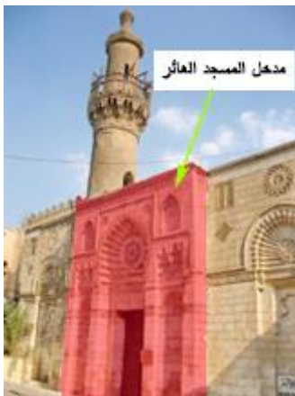
Figure No.3-A Entrance to Al-Aqmar Mosque , www.alhadath.net
