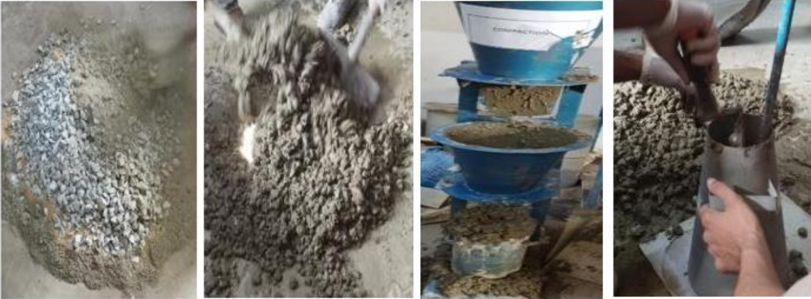
Figure 5: Mixing & Placing of Concrete
