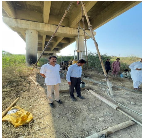
Figure 4: Straight Rotary Drilling Machine on site at (BH-1)
