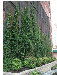
Fig 4: Continuous Living Wall
